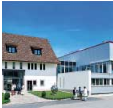
Technology Center, Binzen (Germany)
