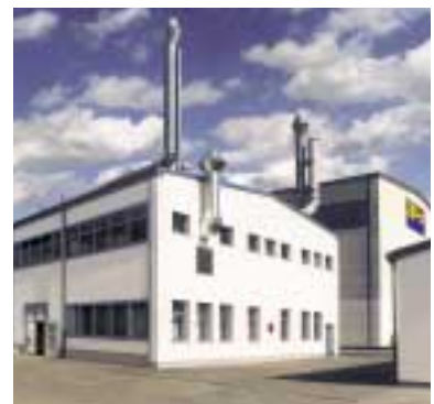
Contract manufacturing facility, IPC Dresden (Germany)
